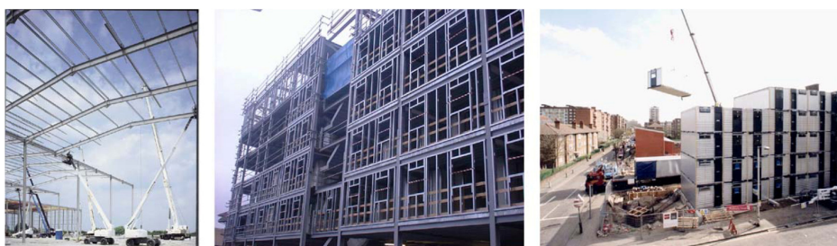
Fig. 3. Prefabricated linear elements, infill panels and complete modules.
