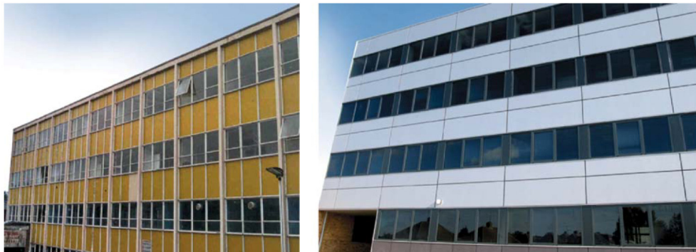
Fig. 7. Before and after over-cladding.
